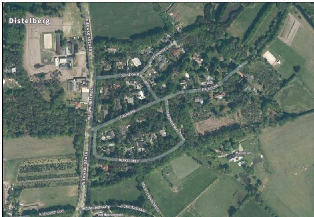
Luchtfoto Distelberg (bron: PDOK Viewer)
